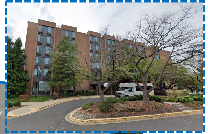
6-story Senior Living Building
